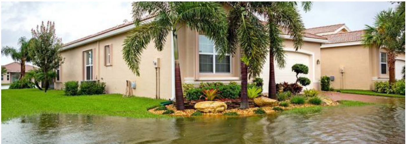
Image 01. A house is surrounded by flooding waters. (Source: ctpost.com).
